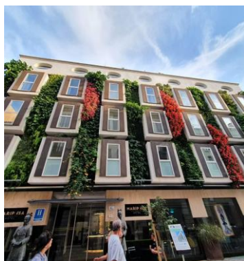
Figure 21: Vertical Garden installed in Malaga
